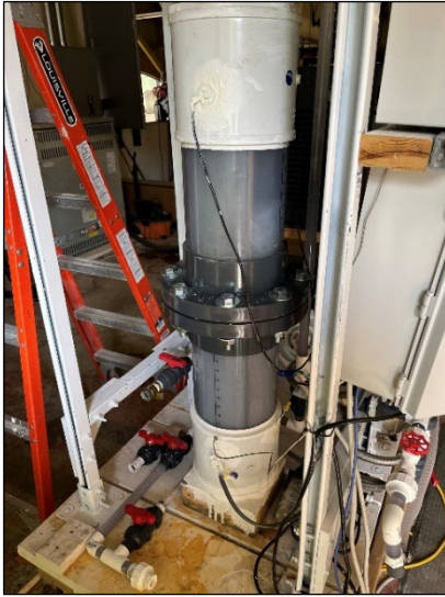
Aggressive boil of brine at at low temperature and deep vacuum per pictures to the right.
